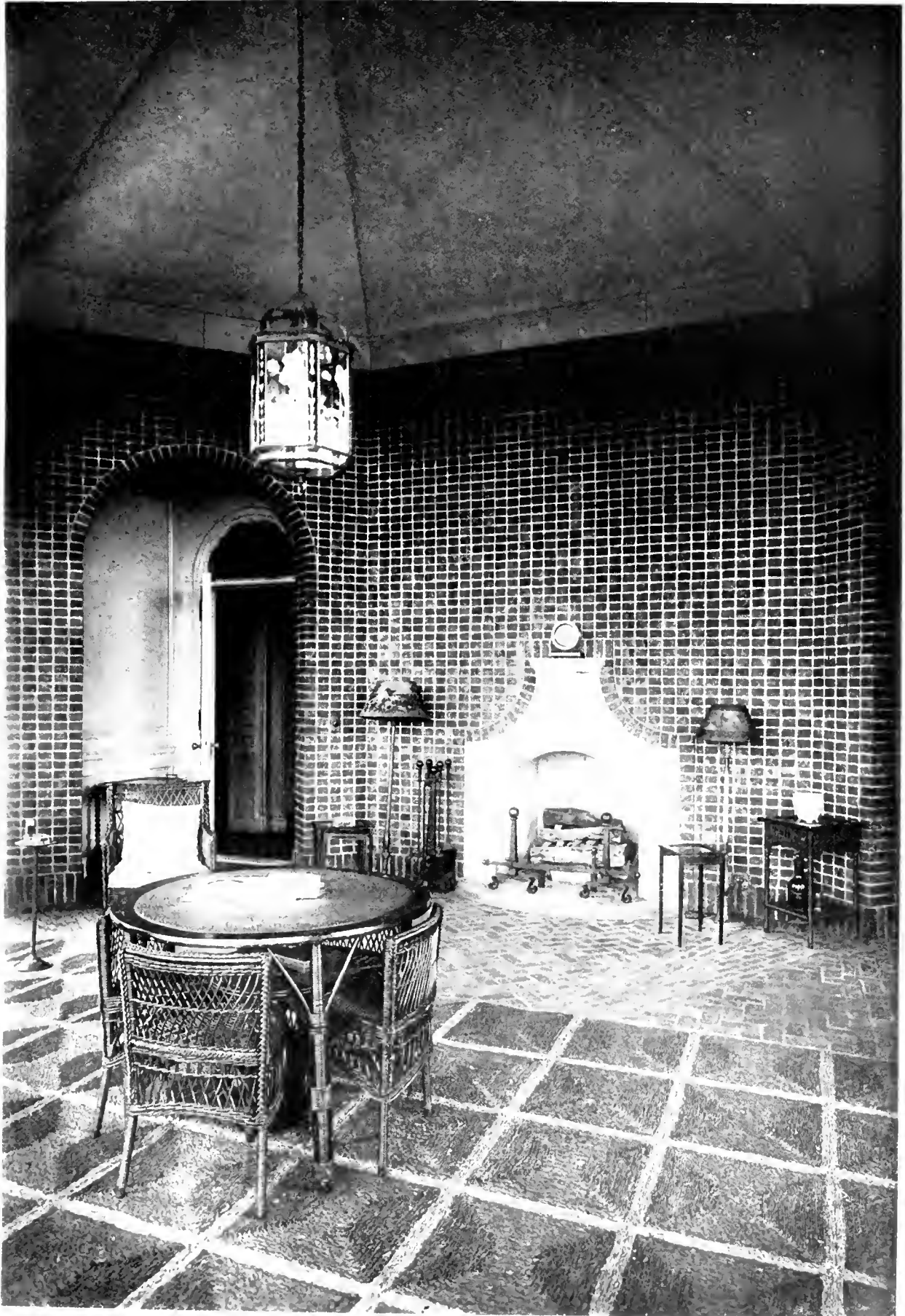
HOUSE OF JAMES J. HILL, OLD WESTBURY, L. I., N. Y. WALKER & GILLETTE, ARCHITECTS
